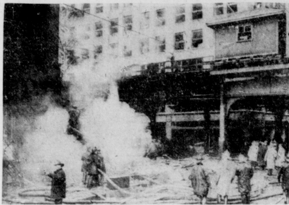
The total remains of a three-story building in Chicago's downtown district is a pile of rubble. The building was leveled by explosions attributed to an accumulation of gas. At least two persons are dead and over 30 injured as a result of the blast which shattered windows and damaged nearby buildings. Property damage is estimated at $1,000,000. (NEA Telephoto).
