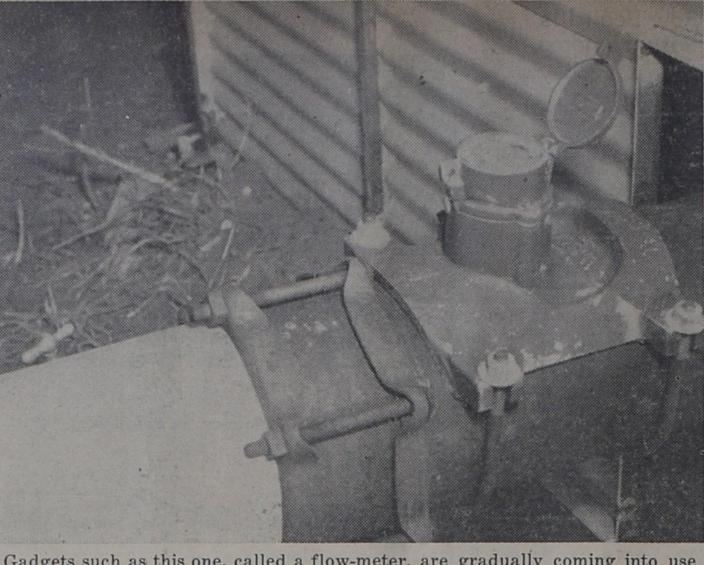
Gadgets such as this one, called a flow-meter, are gradually coming into use to measure exactly the amount of water pumped by a well. This one is on the farm of Walter Kaltwasser in the Oklahoma Lane community.
