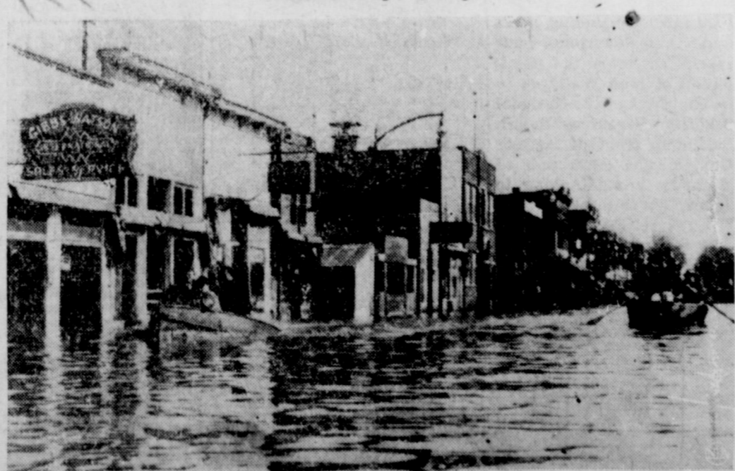
Traffic on Missouri Valley's main street is restricted to motor and rowboats in Missouri Valley, Iowa. The boats ply back and forth removing goods and merchandise from the flooded stores and homes. (NEA Telephoto)
