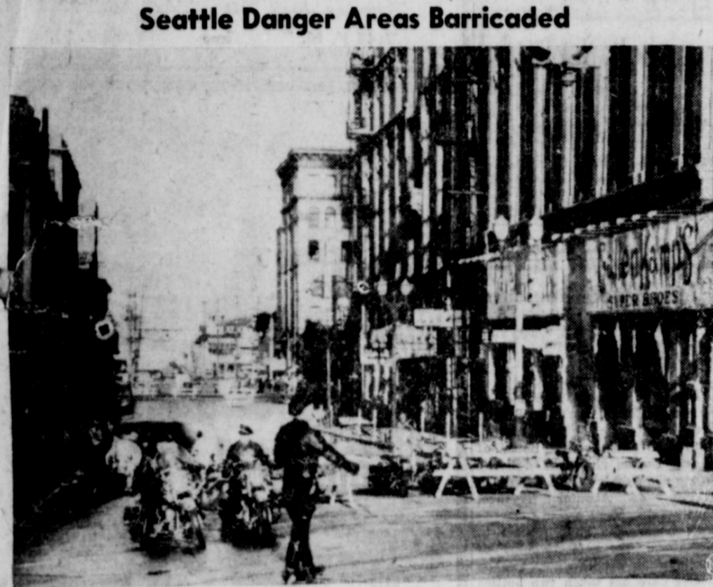
One of the busiest sections of downtown Seattle appears deserted as police barricaded danger areas. The earthquake which was felt throughout the northwest part of the United States made many of the buildings in the city unsafe, and they are being checked before tenants return. (NEA Telephoto.)
