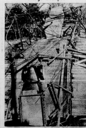
A coal truck hangs perilously from a tangle of wood and on a major construction project steel girders of what was once a bridge over a canal near Little Falls, New Jersey. Another car, not so fortunate, dropped into the canal when the bridge collapsed under the weight of three trucks on the span at the same time. In rear is trailor of the truck-trailor that almost reached solday by spokesmen for El Paso Labor Unions that wage rates were too low for the viaduet project, (NEA Telephoto.)
