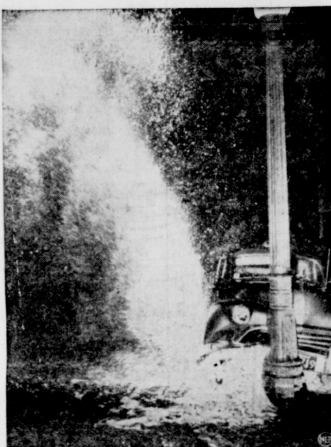
OLD FAITHFUL —A spectacular geyser of water resulted when this auto skidded on car tracks and knocked over a fire hydrant at Charlestown, Mass. The driver emerged unhurt.
