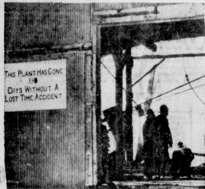
ACCIDENTS WILL HAPPEN —Firemen (right) inspect one of four buildings wrecked when fire swept the Virginia-Carolina Chemical Corporation plant in St. Bernard, O., suburb of Cincinnati. As the sign (left) shows, luck was not with the company on its 100th day. (NEA Telephoto).
