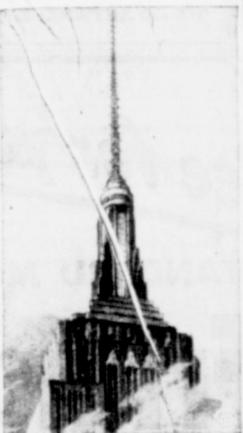
TV TOP—This is an architect's drawing of the new 217-foot multiple television tower being built atop the Empire State building in New York City. The tower, scheduled for completion by the end of the year, brings the overall height of the building up to 1467 feet.
