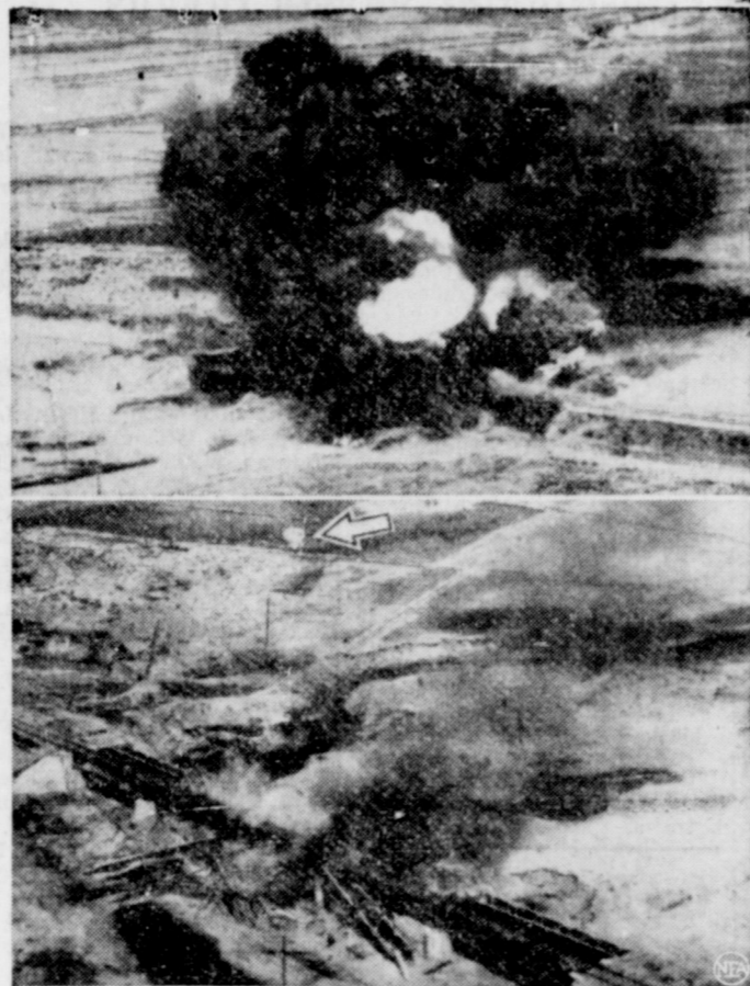
END OF THE LINE —It was "No Trains Today" on this North Korean railroad after Far East Air Force planes clobbered it with parachuted fragmentation bombs. Upper picture shows a direct hit smashing half the railroad bridge. In lower picture, arrow indicates second para-frag bomb descending toward the undamaged part of the bridge. (U. S. Air Force photo from NEA.)
