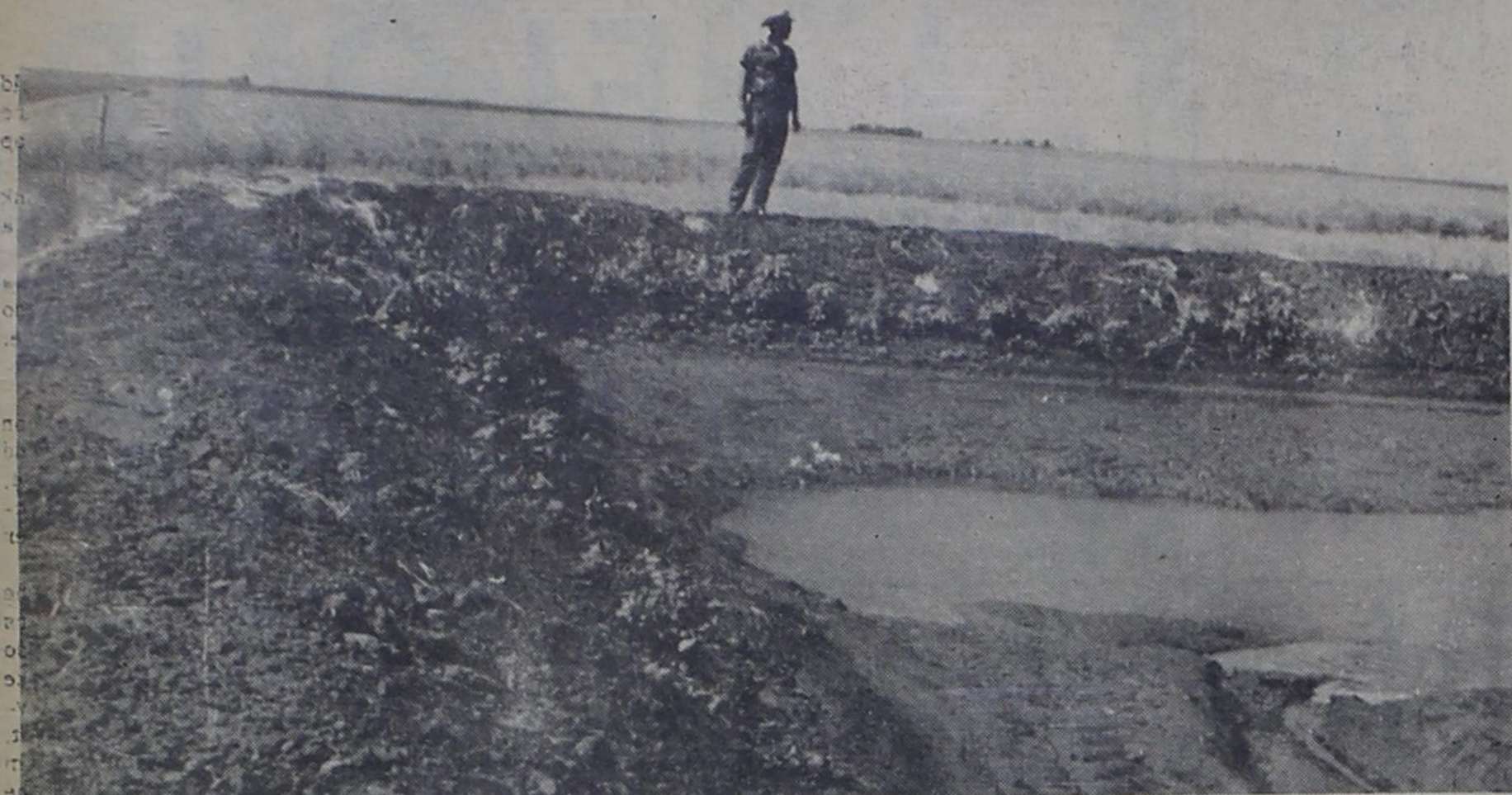
AN EXCELLENT means of curbing tallwater waste is the "low profile" tank, such as the one shown, which is located on the A. L. Hartzog farm south of Bovina. The tank is low
