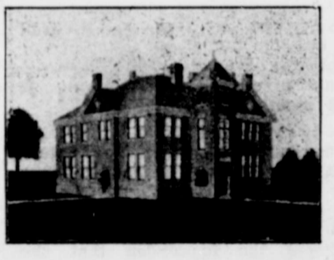
Merkel Public School Building
