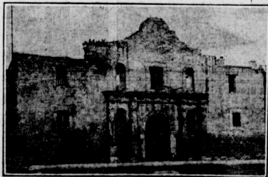
Alamo building as it appears two centuries after erection. The walls are four feet thick and of solid masonry. Bodies of the Alamo defenders were burned in front of this building by order of Santa Anna, Mexican general.
