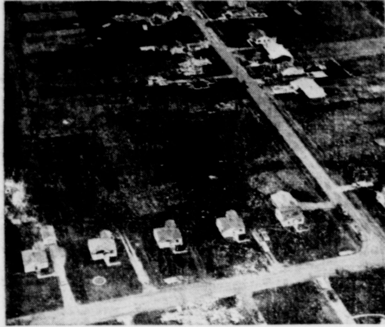
ERRATIC TRAIL left by the twister which hit Flint, Mich., on May 12, 1956 is typical of tornadoes as the funnel weaves and bobs over the landscape, generally in a southwest to northeast direction. Civil defense rescue squads, trained to dig persons out of bombed-out buildings in wartime, find their training equally useful in this type of disaster. (Flint Journal Photo by Russ Scott)
