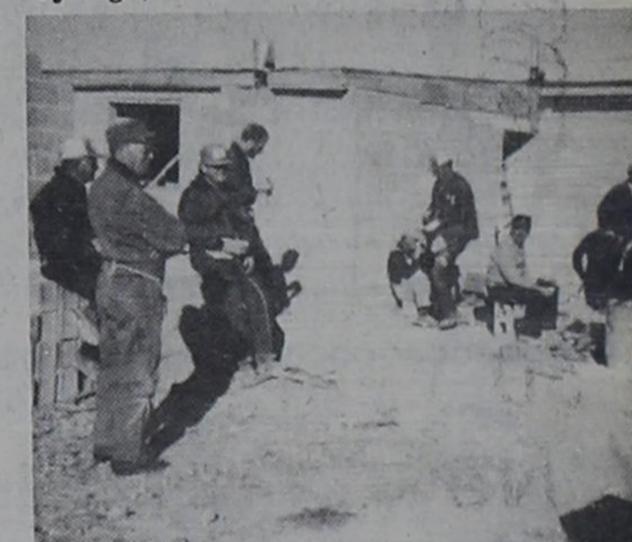
MEN IN THE GROUP are shown taking a break from construction work on a dormitory.
