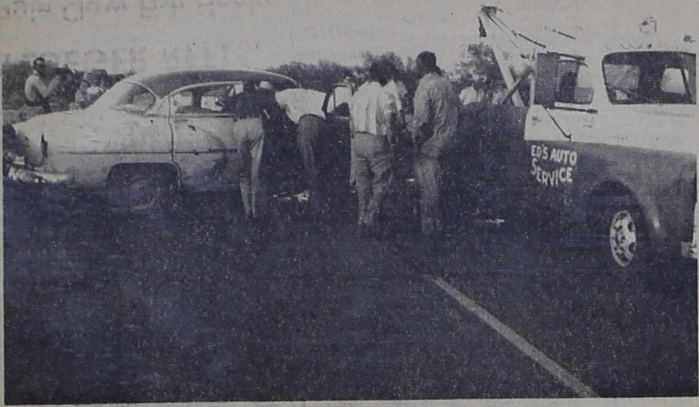
STAYED ON BRIDGE---Though the car in Monday's wreck struck two guard posts before hitting the bridge railing, it stayed on the bridge after the impact. This picture was made looking east. The car, a '54 model Chevrolet, was going west. An Ed's Auto Service wrecker is in right foreground.
