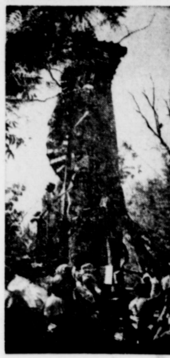
The 44' tall swamp tree slide on Skull Island at Six Flags Over Texas is built around what once was a fire escape at a dormitory at the University of Texas. Guests climb the spiral staircase around the outside of the tree and slide down the long corkscrew-type slide inside.
