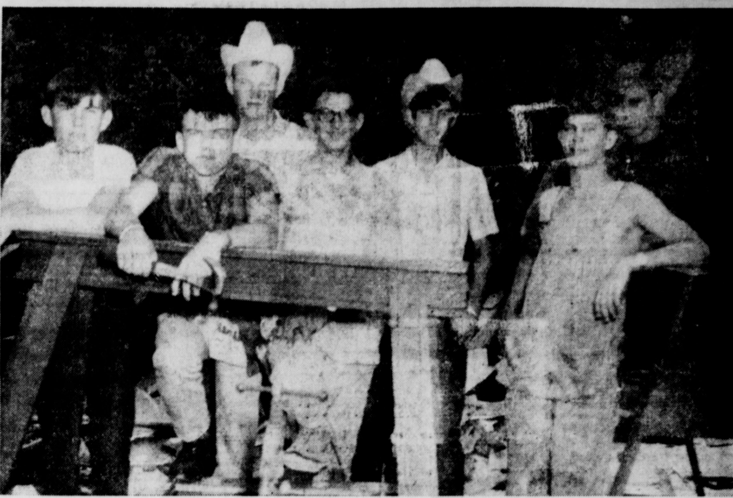
TIME OUT FROM WORK — MHS Shop Boys agree it's time for a "break" from house building. Relaxed and "ready to go back to work" on the new home going up for Arthur Moore are,
