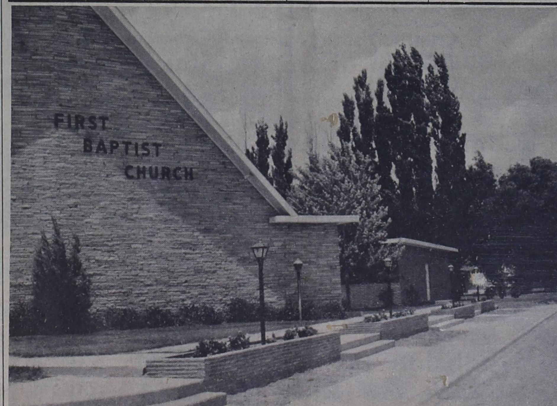
CHURCH IMPROVEMENTS -- Recently completed were these exterior improvements at First Baptist Church of Bovina on Third Street. The flower boxes, front and right, were installed as were the lights in each box, the steps and walk.
