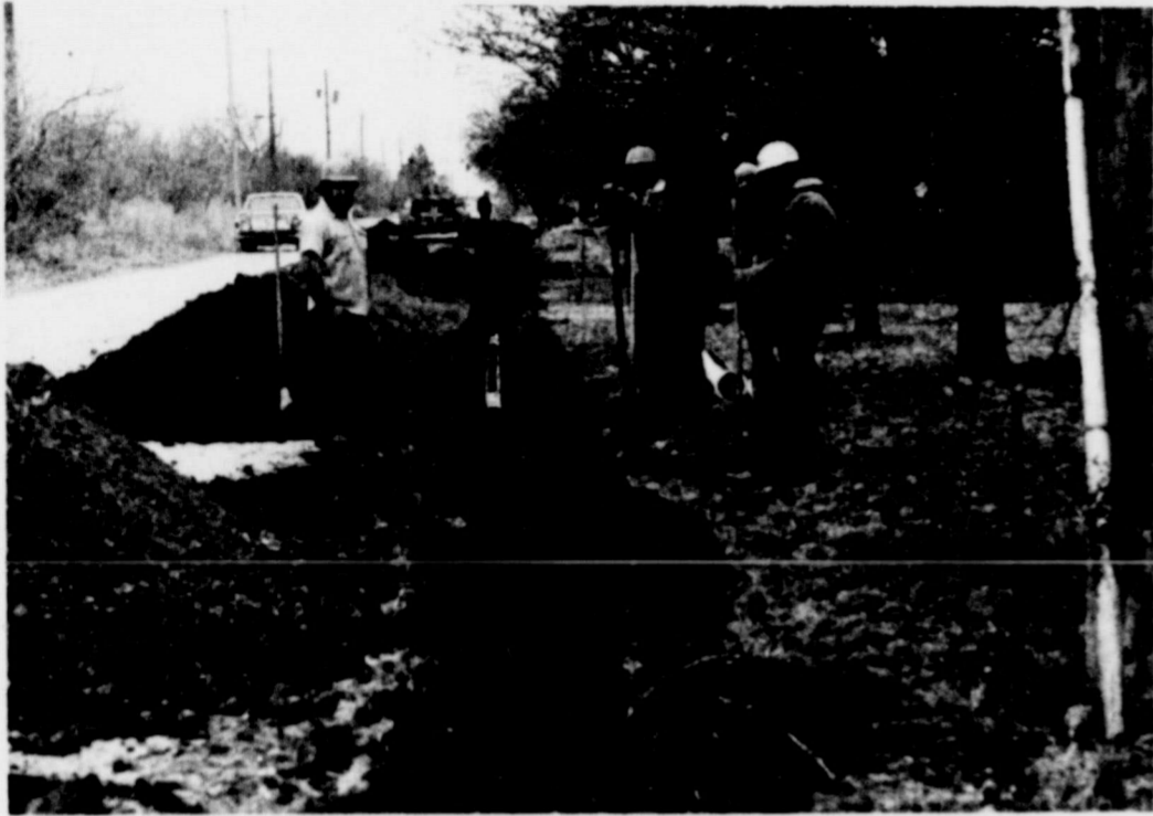
Water project in progress at the intersection of West and Haynes Streets.
