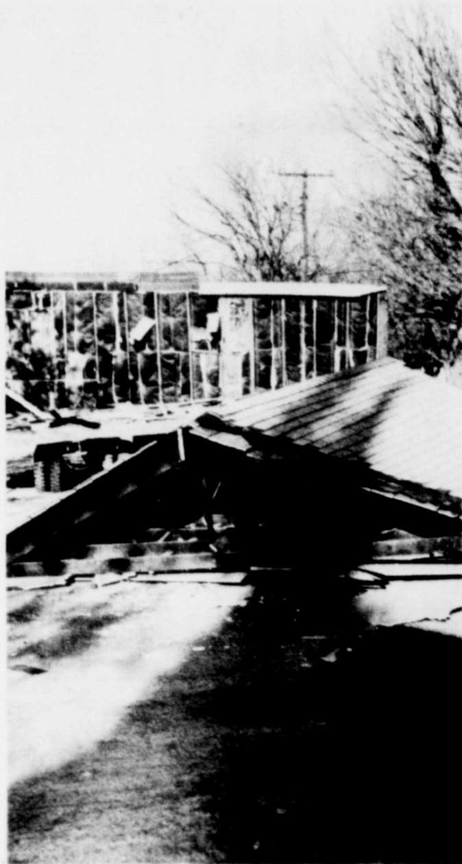
It's not a Tornado! These two halves started as one building, the roof came off while workmen were trying to move the house. (Staff photo by Glenn Richards)
