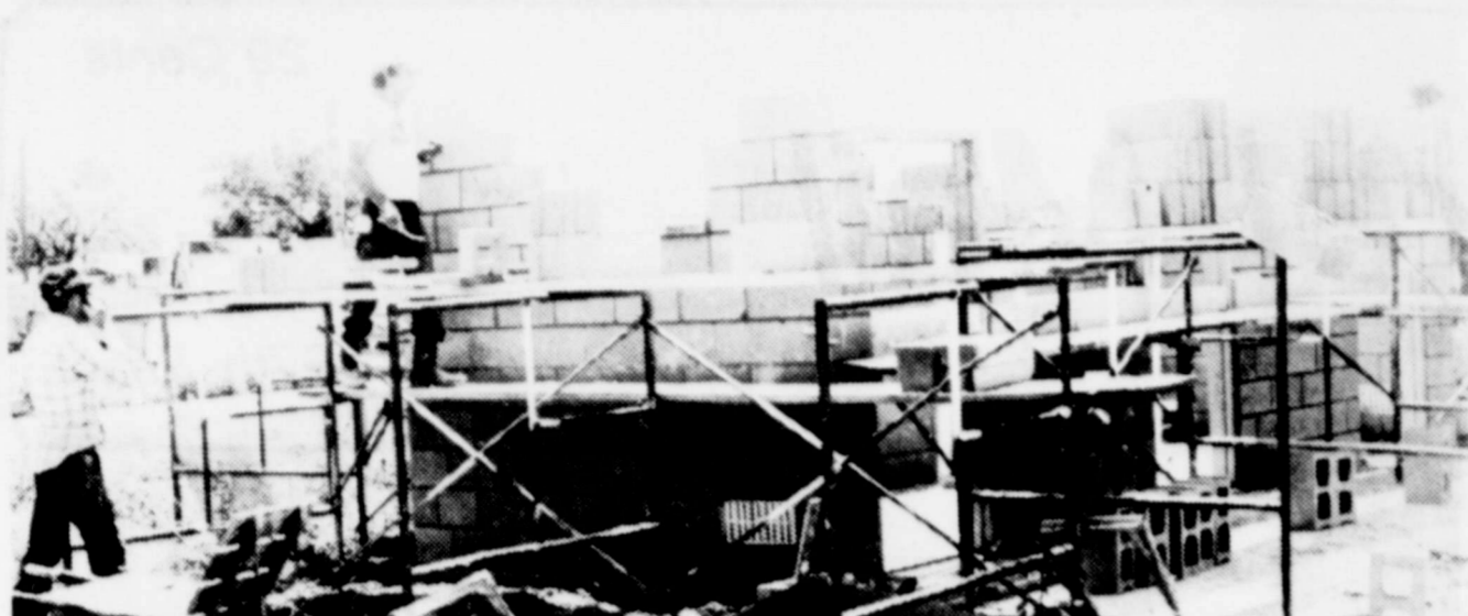
Restroom facilities for the new City Park were being constructed Monday. The park is being built South of the Interstate Access road and West of Circle A Western Wear. [Staff photo]
