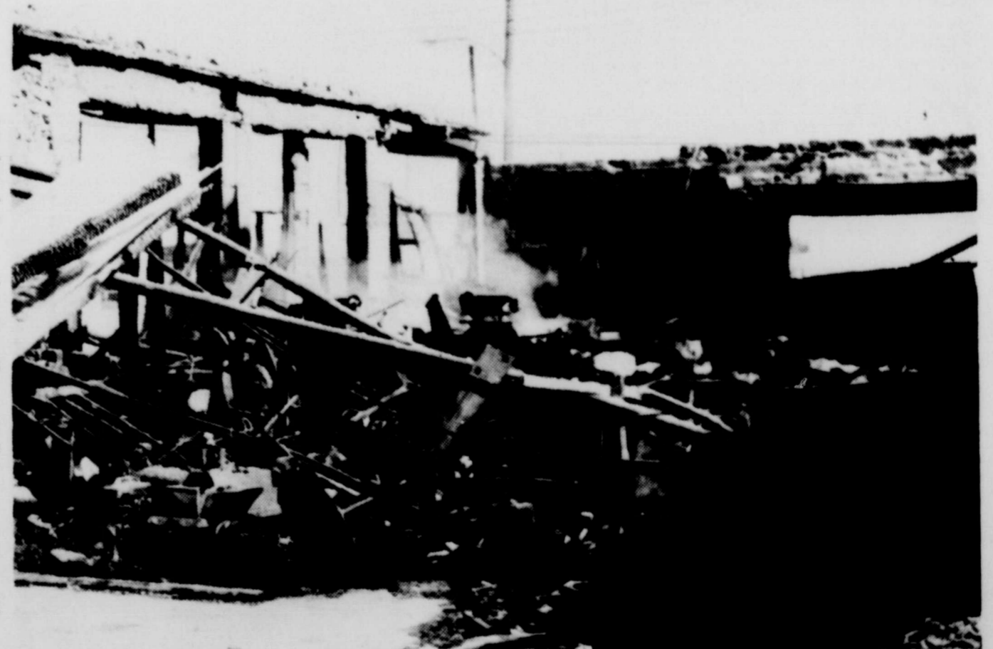
§ Two local businesses were destroyed as a fire broke out at 4 a.m. Monday. The office and shop of Consolidated Plumbing and Browne Enterprises were gutted by the early morning fire. Local
