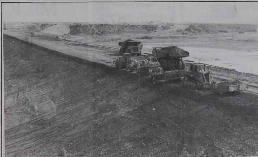
A CLOSER view of the dam shows some of the heavy equipment that is being used to haul in the more than six and a half million cubic yard of earth used in the construction of the project. (Photo by John Cordsen)
