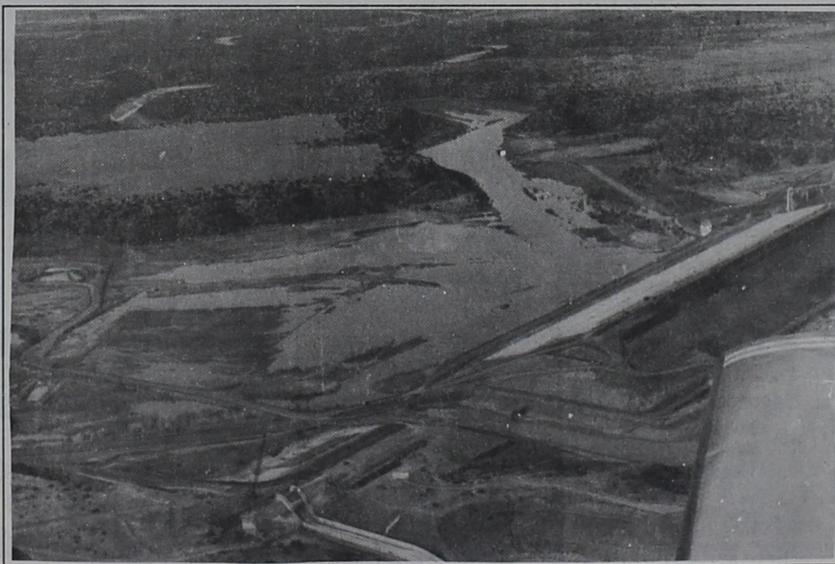
A BIRDS-EYE look at Lake Allen Henry dam south of Post shows how close to completion construction on the 3,300 foot wide dam is from being done. Note the opening to the bottom of the photo, this hole alone will take over one million cubic yards of dirt to fill. (Photo by John Cordsen)
