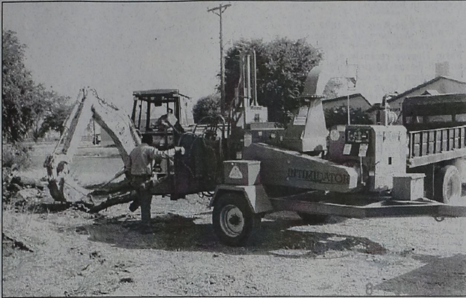
RIPPIN' AND CHIPPIN'.... City workers use the new wood chipper to clear limbs and brush. Bovina city manager Ernest Terry and Friona city manager Paula Wilson cooperated on a grant program that brought the two cities this 18" wood chipper. A schedule will be established for use of the chipper in each city. photo by Ernest Terry
