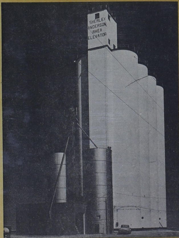
SHERLEY-ANDERSON RHEA ELEVATOR JOE ALLEN
