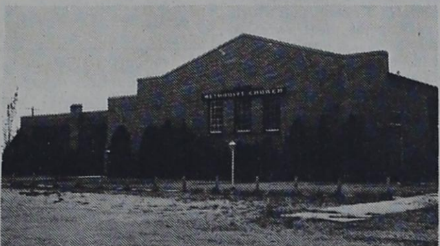
Oklahoma Lane Methodist Church
