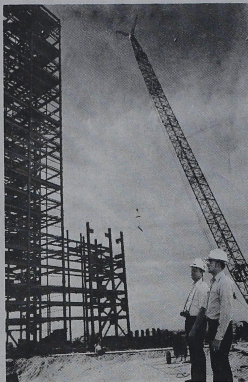
LOOKING OVER Southwestern Public Service Company's Tolk Station construction site
