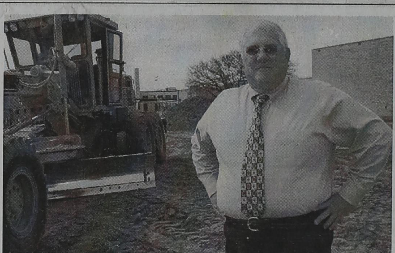
Post ISD Superintendent Marlin Marcum stands in the area where construction recently began on the new school cafeteria. (Staff photo by Tim Burnett)
