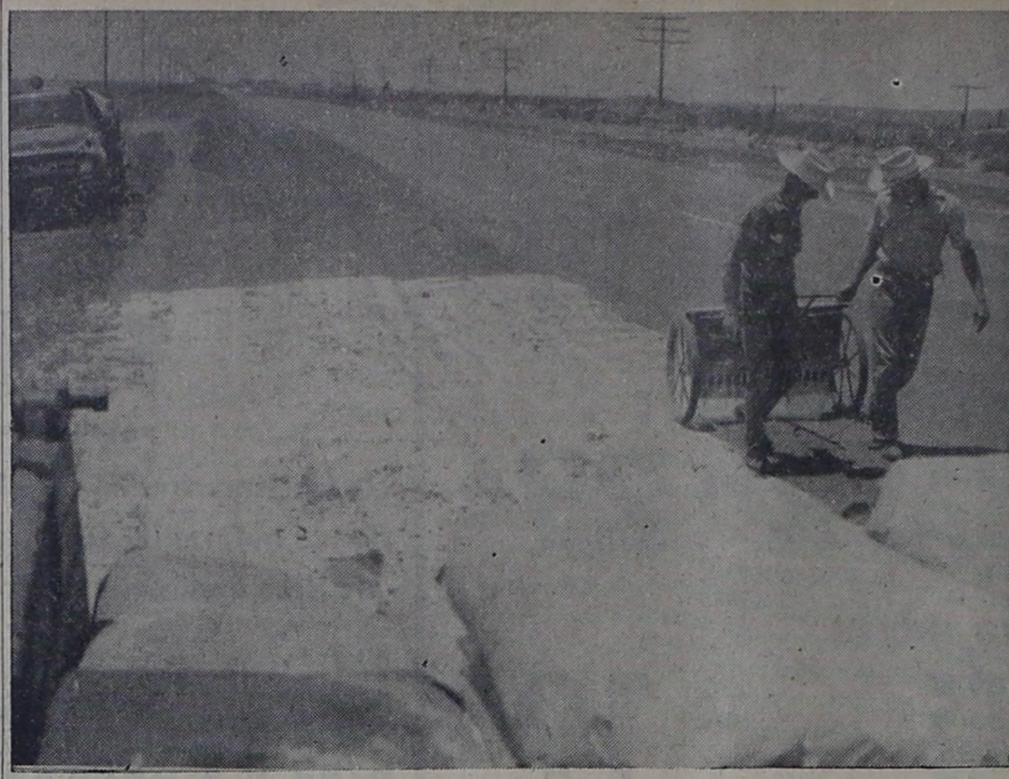
Parmer County's employees of the Texas Highway Department got their bindweed control work underway last week. Here they are making application on an infestation near Lariat in the southern part of the county. Running the spreader are Bobby Englant and Alfred Haney.
