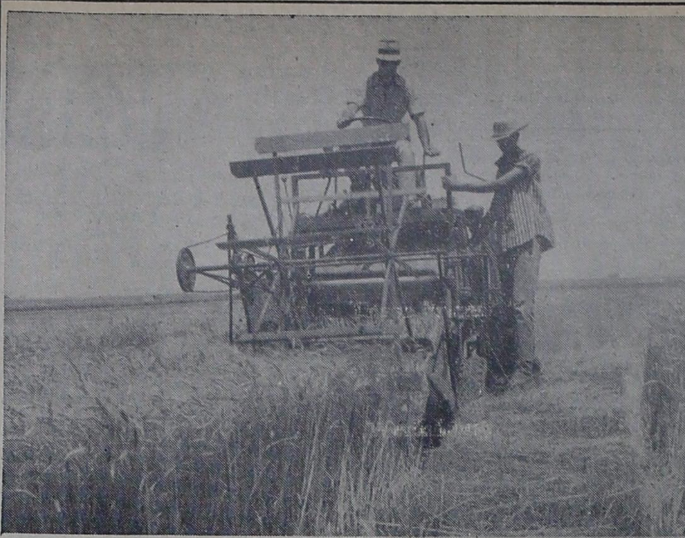
This specially constructed four-foot combine was used to harvest check plots of wheat on the Walter Kaltwasser farm in the Oklahoma Lane community. Tests conducted by Al Pope of the Amarillo Experiment Station are intended to show responses to fertilizer and other practices under varying conditions.
