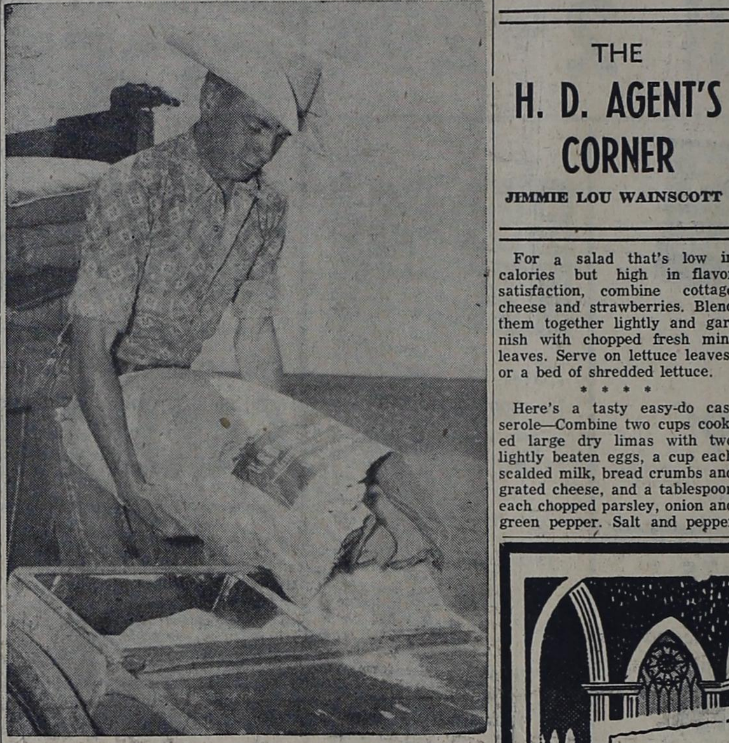
Leon Richards, Highway Department employee, empties a sack of soil sterilant into a waiting spreader. Borascu is the chemical being used by the state to control bindweed.
