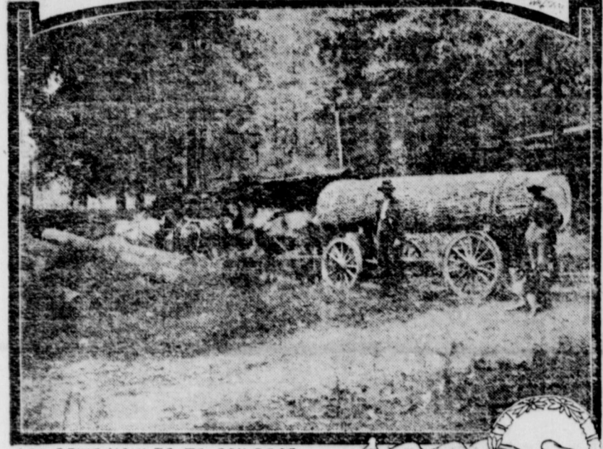
LOG BEING HAULED TO RAILROAD
