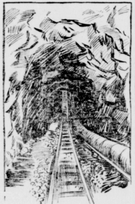
Tunnel Through Which Gunnison River Will Hereafter Rush.
