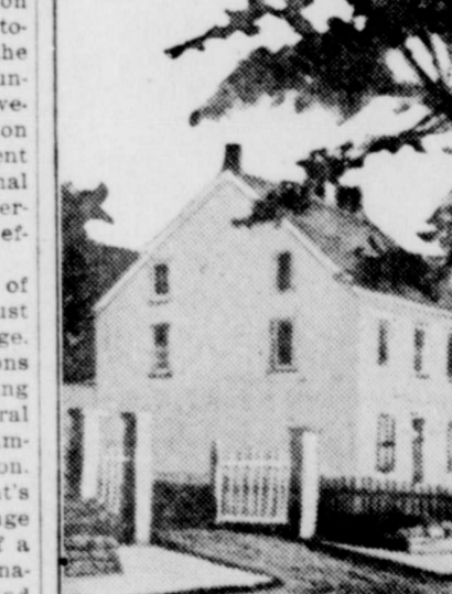
Roxborough School, 1748; Rebuilt 1894.
