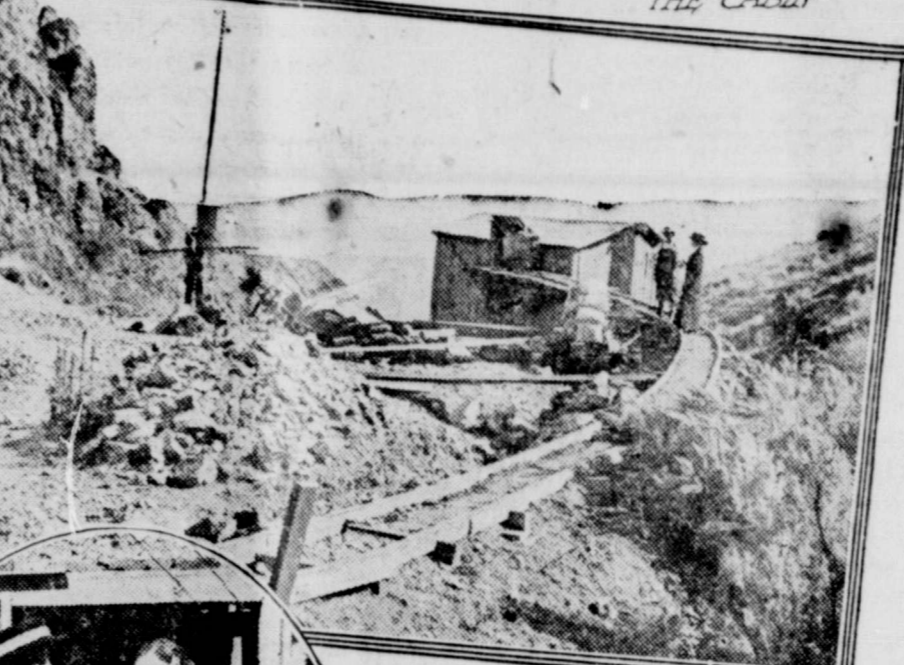
RAILROAD LEADING FROM HINE TO MILL
