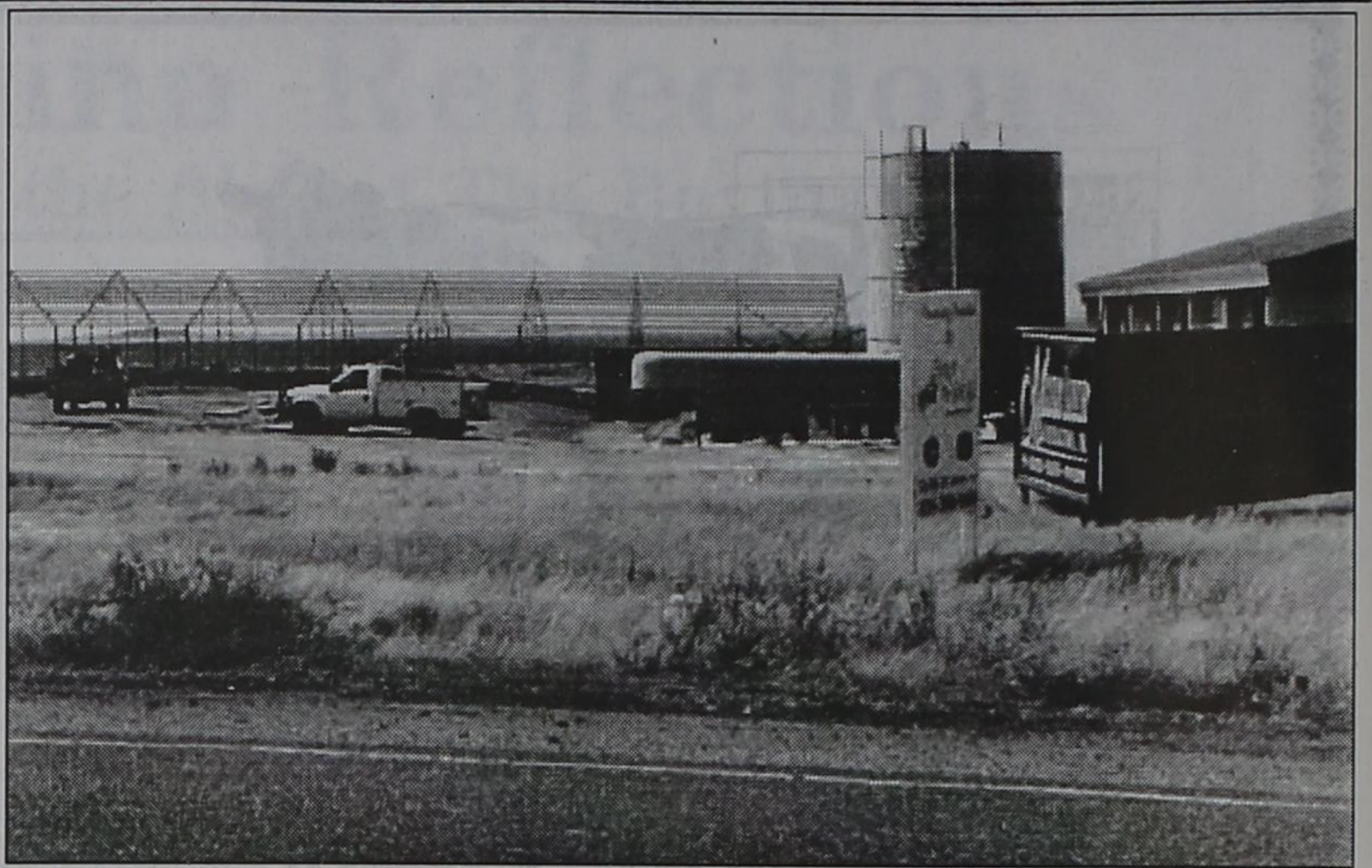
CONSTRUCTION is progressing on the High Plains Dairy located about 6 miles east of Hub on Highway 86. These views are taken looking south from the highway.
