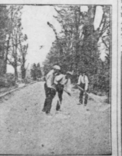
Making Necessary Repairs on Macadam Road.
