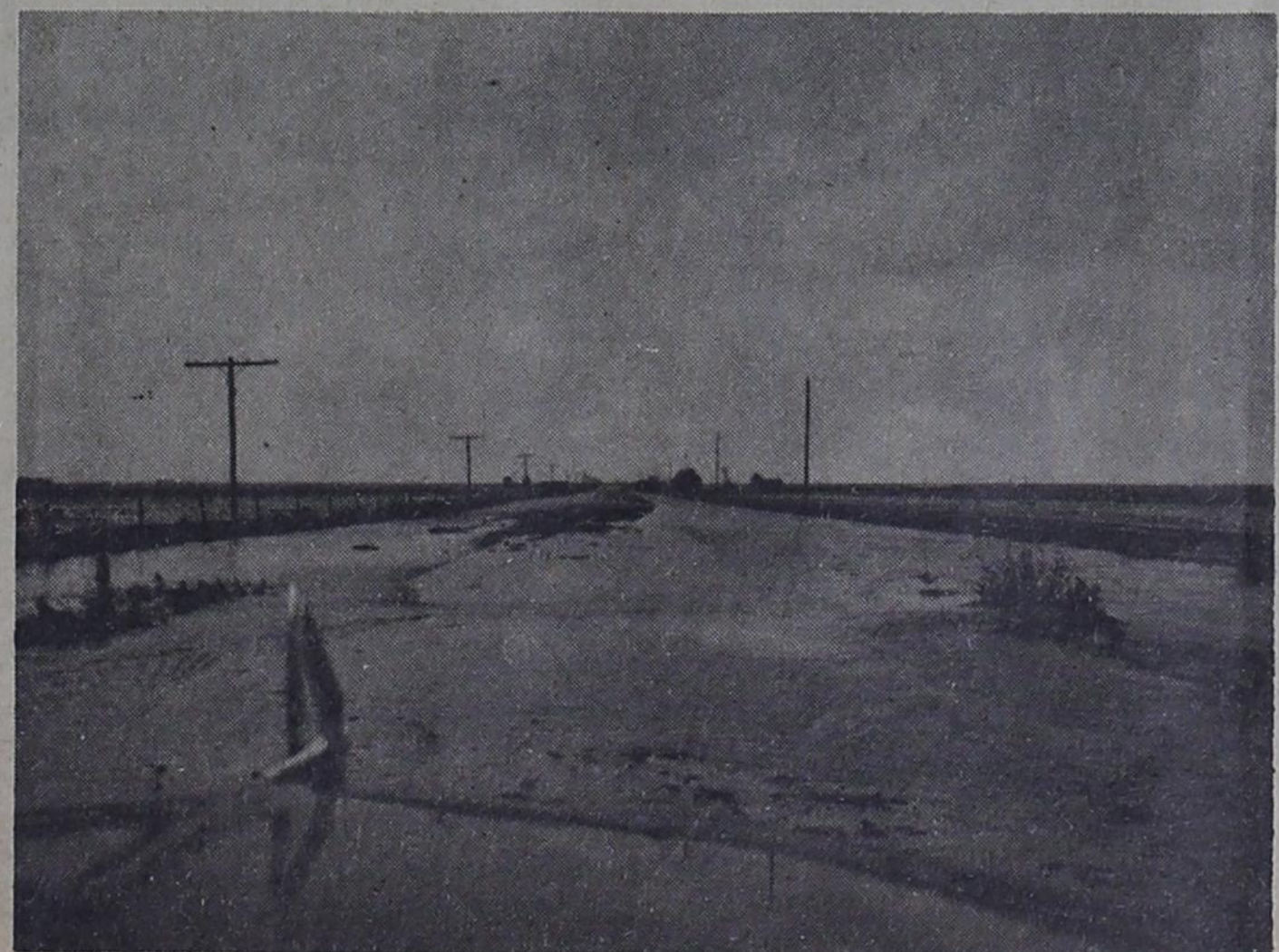
"MUDDY ROAD AHEAD" --A downpour some three miles north of Bovina Friday afternoon brought tremendous amounts of water swishing down Farm Road 1731. This scene is looking north on the FM Road. Ditches on each side of the pavement were swollen out of their banks.
