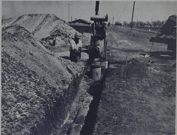
INSTALLING PIPELINE -- An underground concrete pipeline irrigation system is being installed on the Reagan Looney farm two miles southwest of Bovina. The system is designed to conserve irrigation water, Soil Conservationists say. (Photo by Jerry Isbell).
