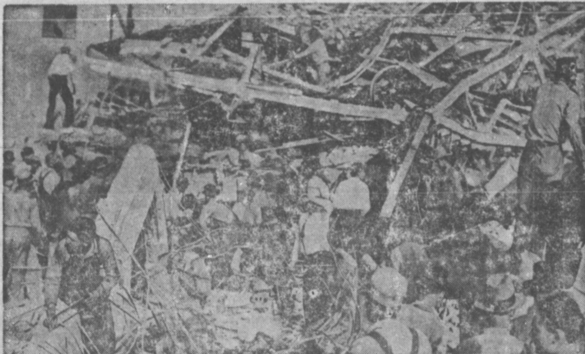
Rescue workers at scene soon after Texas school was blown up, engaged in hazardous task of bringing out the dead.
