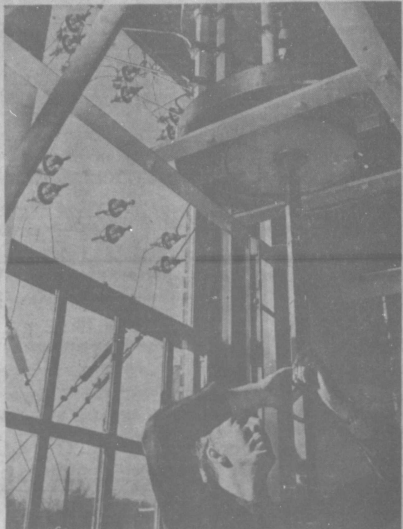
DIRECTING A MESSAGE—Radio operator selecting directional antennas at the Columbia Broadcasting system's international station W2XK. These antennas enable the broadcaster to concentrate the station's power in any given direction.
