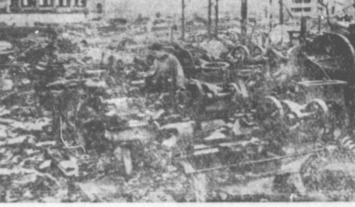
Home as well as factory industrial facilities felt the lash of U. S. air raids, with only the machinery standing in the ashes of this burned-out residential shop in Tokyo.
