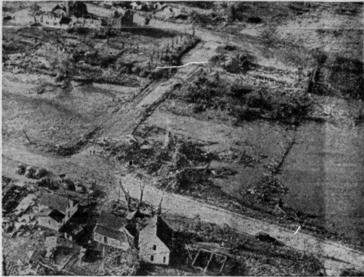
HAVOC IN WAKE OF TWISTER . . . Here's an airview of the extensive damage wrought by tornado which swept through Duncan, Iowa, population 100, recently. There wasn't a house left undamaged by the freak twister which caused one million dollars damage and injury to five persons.
