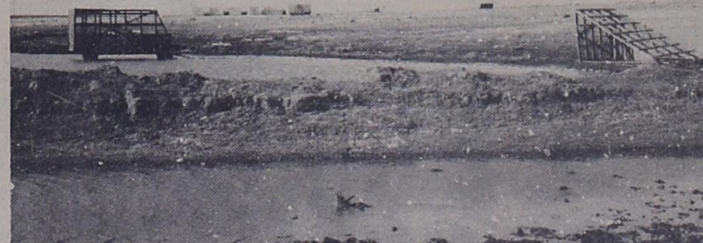
TRAILERS SCATTERED -- Only about five out of 12 trailers on the Lawrence Jamerson place were left in a row, background, where they were anchored after a tornado touched ground east of Bovina Sunday afternoon. Trailers and a mile and a half of irrigation pipe were scattered over the pasture.
