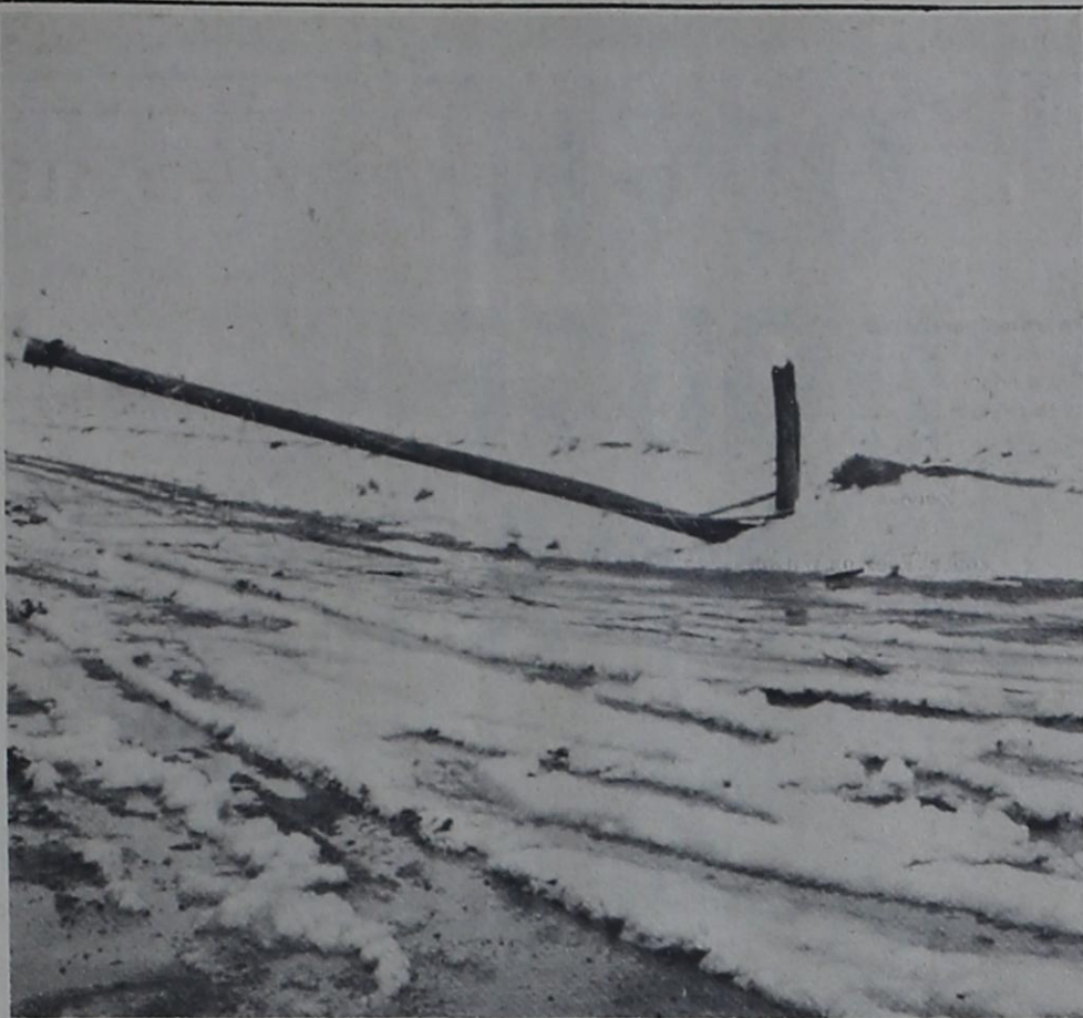
DOWNED POLES... Although Tuesday morning dawned bright and fair, the rural area around Bovina was without electric power as power lines and poles were down over a large area. In one two-mile stretch of Pleasant Hill Highway, only four poles out of over 24 remained upright under the weight of the extremely wet snow. The snow as believed to have been heavier west of town.
