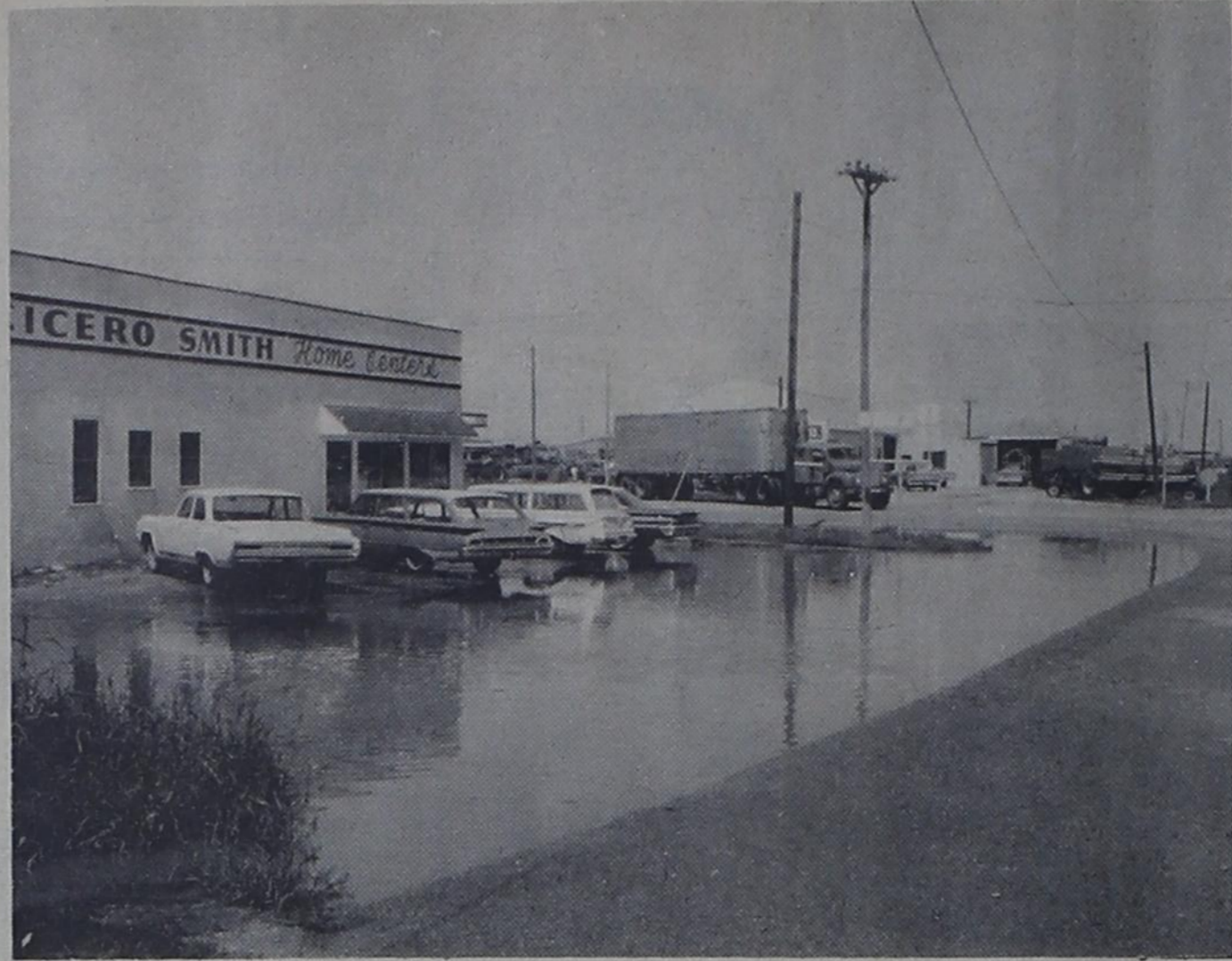
LAKE CICERO -- Lack of proper drainage causes water to stand around Cicero Smith Lumber Co. at the intersection of Highway 60 and Third Street following a rain. This was the scene around the business Monday after Sunday night's rain which totaled approximately 1.5 inches.
