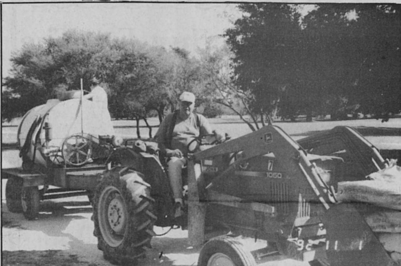
Hoagy Nelson, on front end loader, and Treg Mitchell spread Calcium Chloride on cart paths for dust control.
