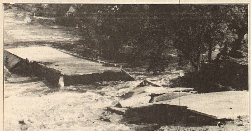
The newly constructed bridge at Pinto Creek Crossing was washed away Thursday morning. Photo by Wes Robinson
