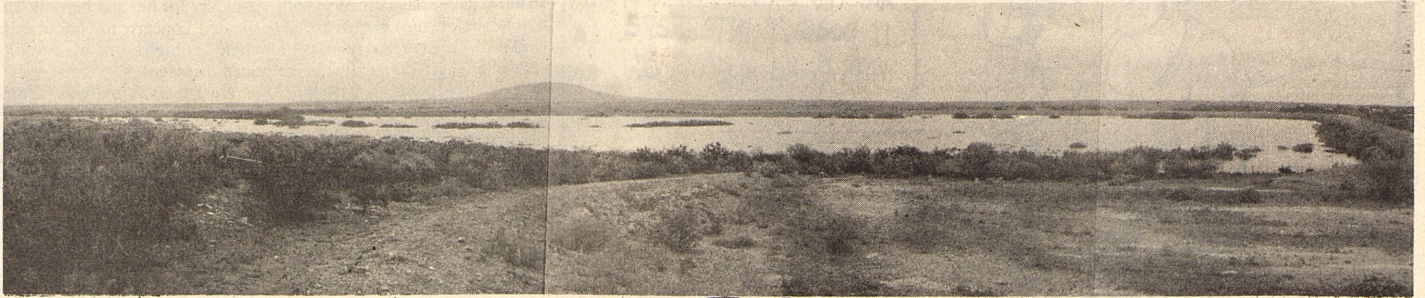
Flood damage in Kinney County could have been worse last week, but two dams north of Brackettville helped slow down the raging water, according to District Conservationist James Crumley. Brackett News Photo by Wes Robinson
