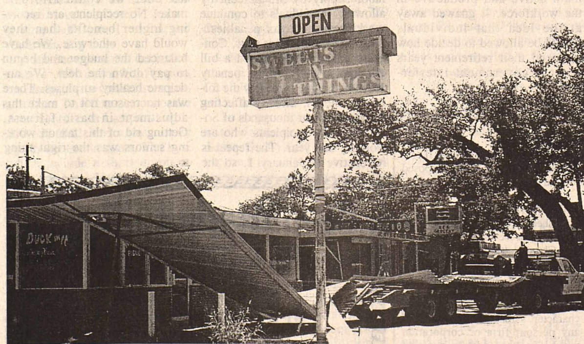
Work crews will tear down these buildings to make room for a 4,000 square foot building that will house a new and improved Pico Store, according to Rick Alvarado, manager. The new store also will bring more jobs to the area.
