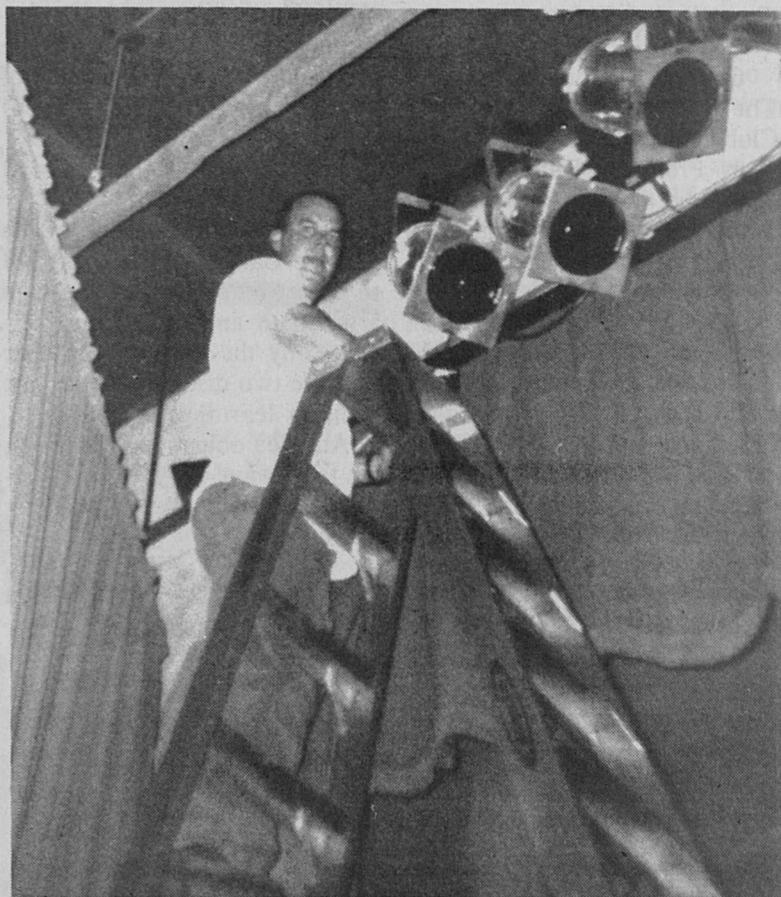
Ben Goodchild, of Superior Decorating, installing new curtains at Post Theater
