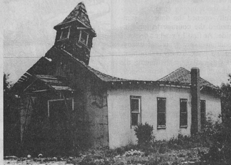
Pictured above Mt. Gilead Baptist Church. The building was moved from Fort Clark in 1916 by the Seminole congregation.
