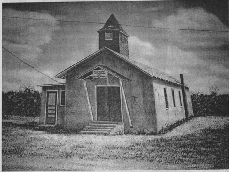
Painting of Mt. Gilead Church by Charles Becker, before it fell into disrepair, hangs in the Filippone Building.
